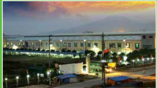
Second factory: Que Vo Industrial Zone, Bac Ninh province
